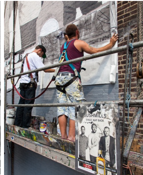
Our painters pouncing a sign space in 2012
